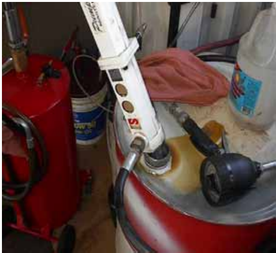
No bung adaptor Open exposure to the elements
